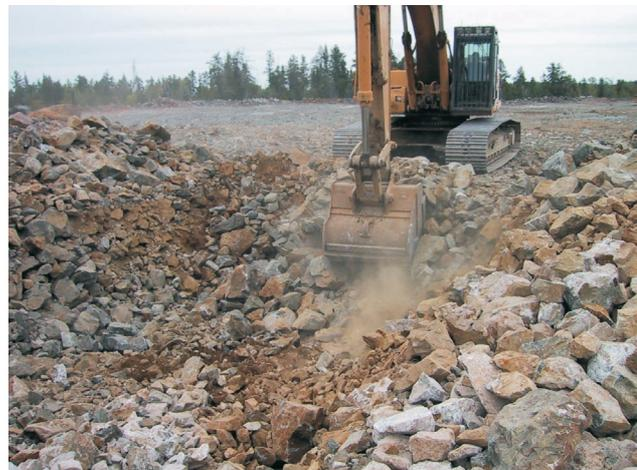
FIG 11 - Test pit excavation at Site 2. Large cobble to boulder sized particles typical of waste rock with small fraction of fine particles in matrix material.
